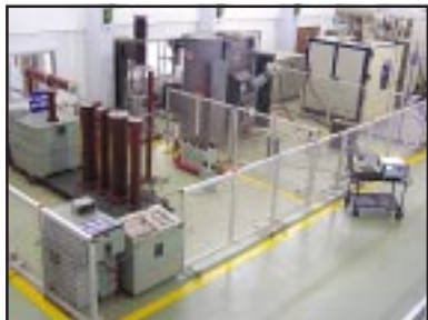
A view of HV capacitor test-bay
