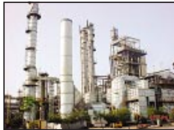
Waste Heat Boiler in Ammonia Plant
