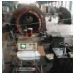
Partial Discharge Measurement on Turbo Generator Stator Winding
