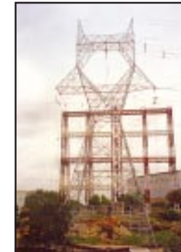
765 kV S/C type 'D' tower
