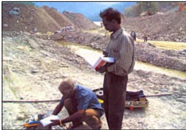
Soil Resistivity Measurements Underway at Teesta Hydro Electric Project Site
