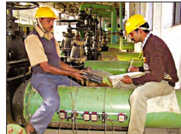
Ultrasonic water flow measurement in progress
