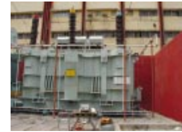
RVM Test on Generator Transformer
